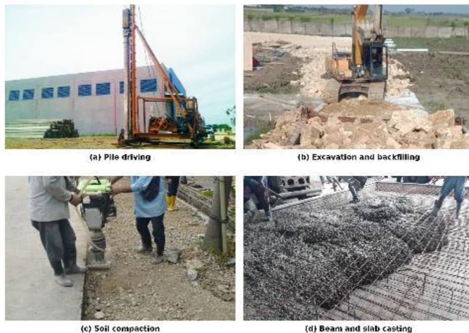
Figure 2: Selected structural activities observed on site. Source: project documentation, 2023
