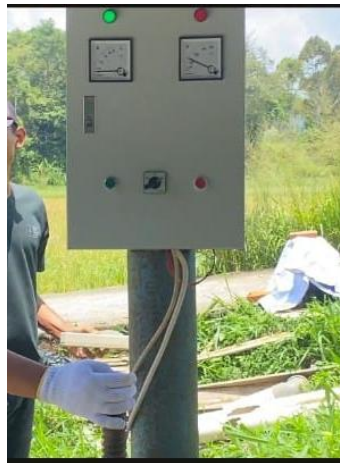
Figure 8: Electrical panel installation
