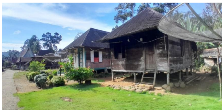
Figure 6. Appearance of A Wooden House (Semi-Permanent) in Nagari Kajai, West Pasaman
