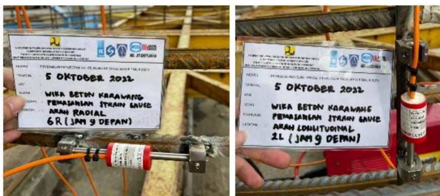
Figure 2. (a) Radial Strain Sensor Placement (b) Longitudinal Strain Sensor Placement
