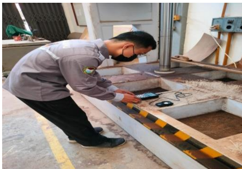
Figure 7. Measurement of air circulation in the ventilation room
