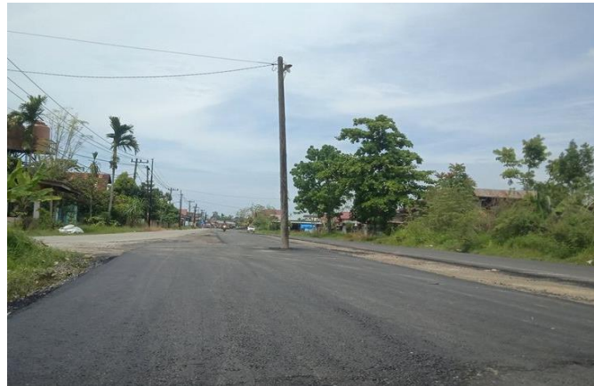
Figure 1. Electric poles are on the road at the Kurao road project, Padang
