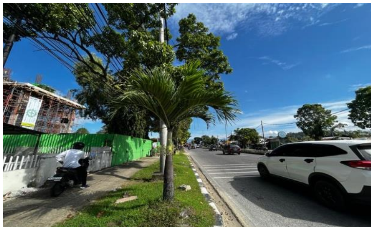
Figure 1. Visual Condition of Khatib Sulaiman Road Section
