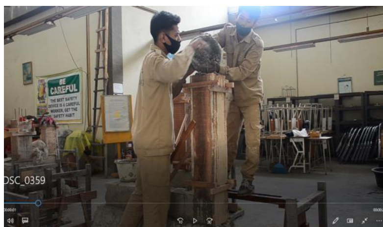
Figure 7 : Column Casting Process
