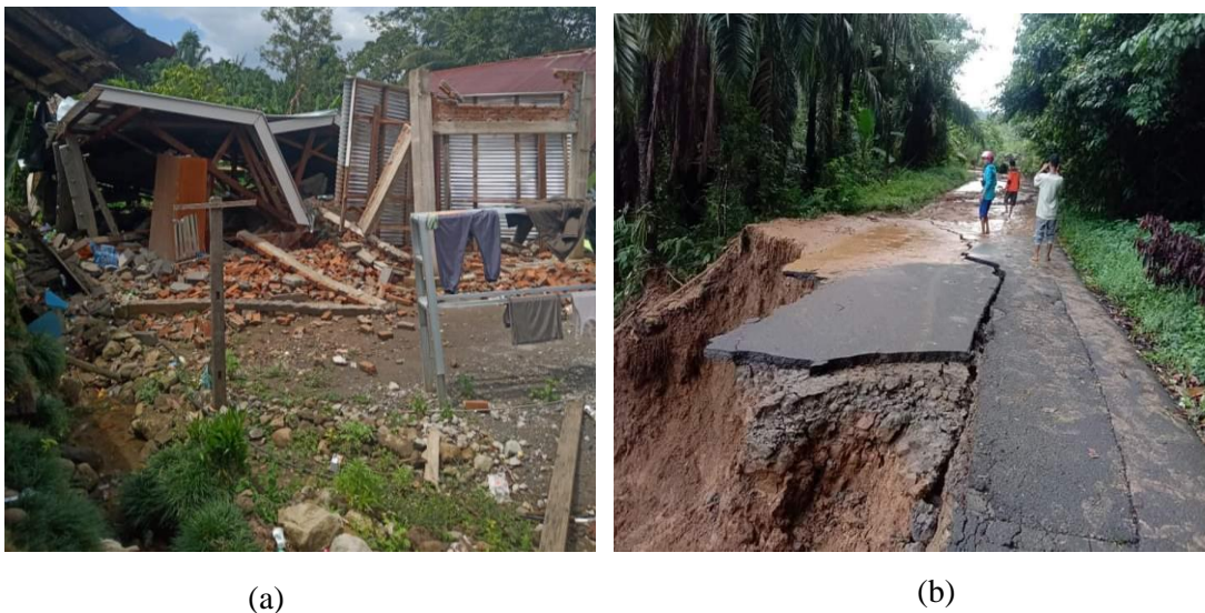
Figure 3. Earthquake Damage (a) House Collapse and (b) Landslides
