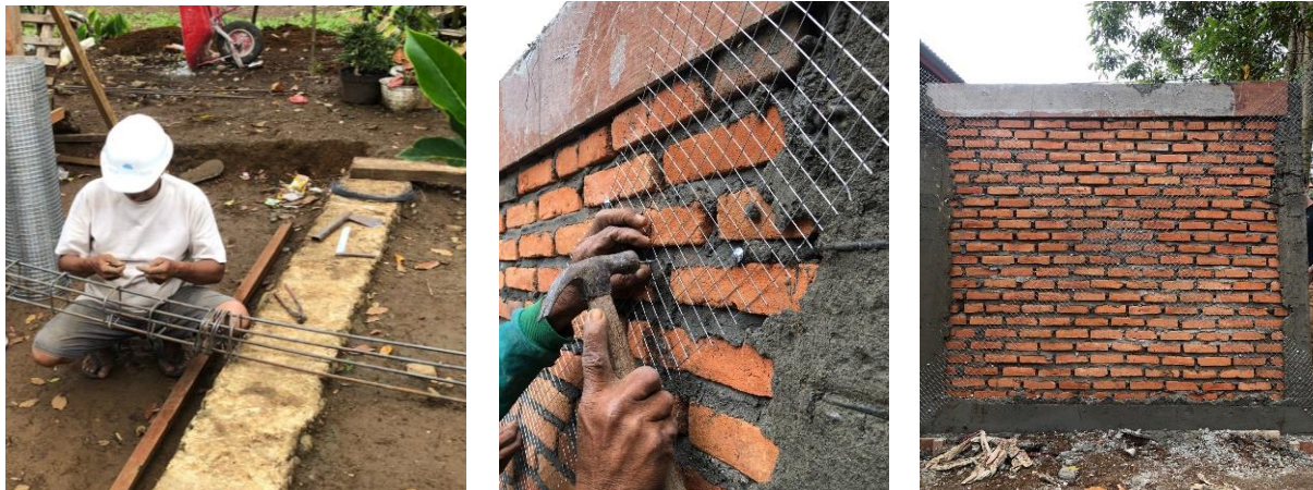
Figure 15. Making Earthquake Friendly House Wall Modeling
