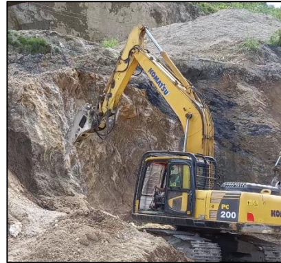
Gambar 4. Excavator Komatsu PC 200-8 M1 (Breaker)
