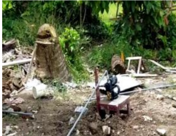
Figure 3: Installation and setup of the water pump.
