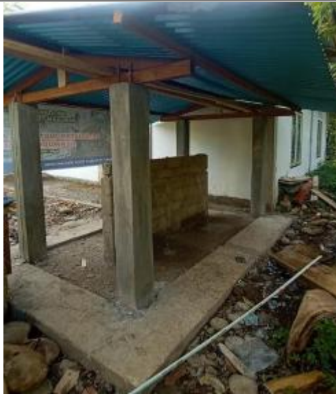
Figure 8: Completed structural form of the ablution facility.
