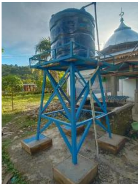
Figure 5: Painted tower, piping installation, and 500 L water tank.
