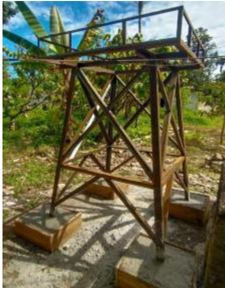
Figure 4: Construction of the water-tank tower.
