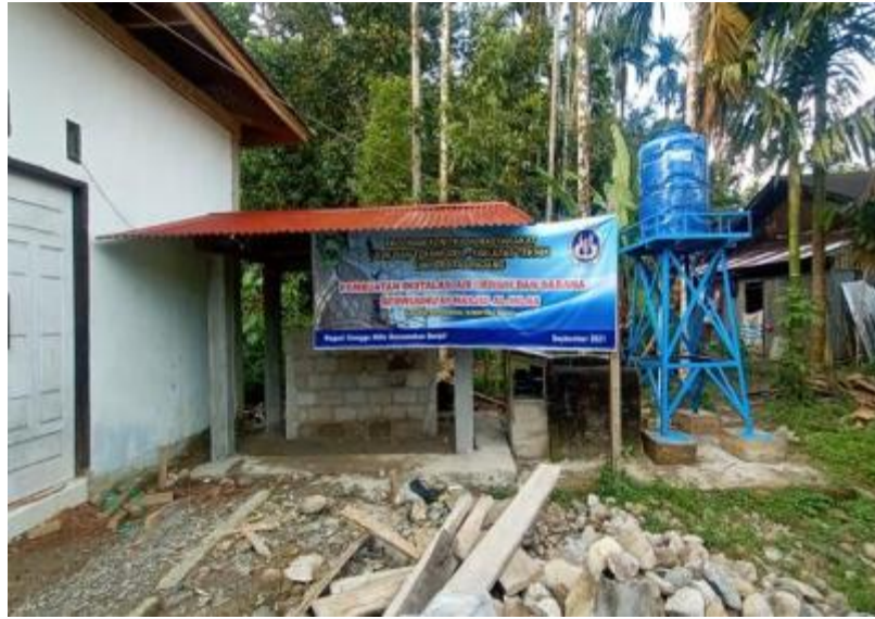
Figure 10: Completed clean-water and ablution facilities at Al-Ikhlas Mosque.
