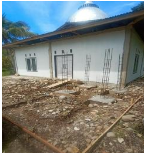
Figure 6: Assembly and casting of reinforced columns.
