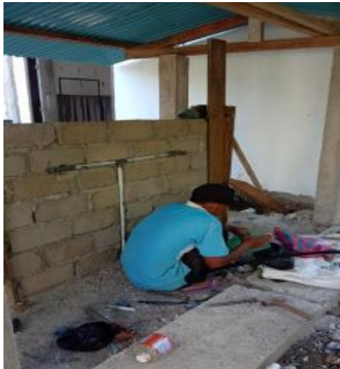
Figure 9: Installation of PVC pipes at the ablution facility.
