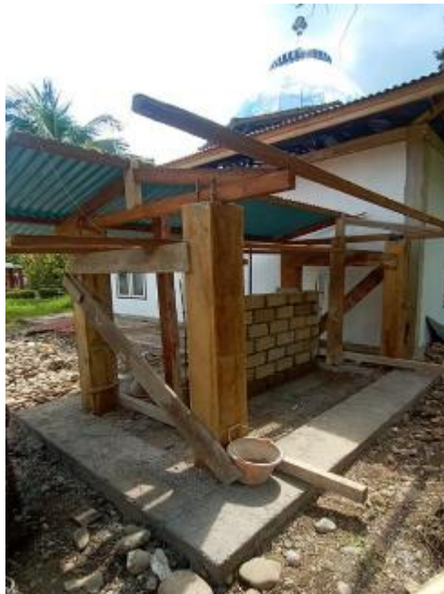
Figure 7: Floor and column work, concrete-block walls, and roof installation.
