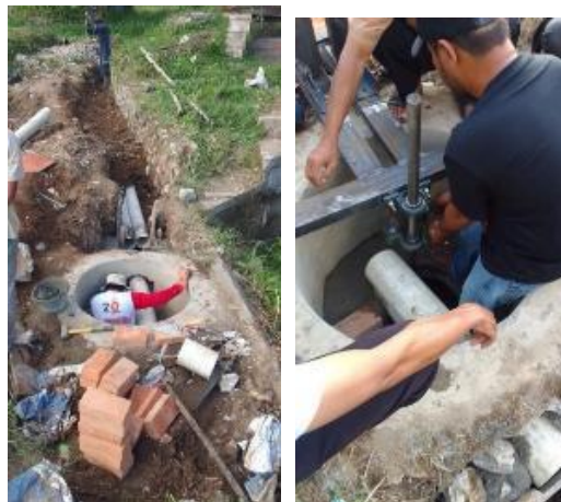
Figure 9: Assembly of Inlet and Outlet Pipes and Installation of Micro-Hydro Power Plant Water Resources Building
