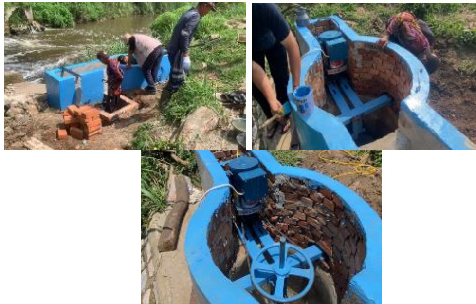
Figure 10: Construction Process of the Micro-Hydro Power Plant
