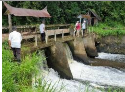
Figure 1: Irrigation Water Control Structure
