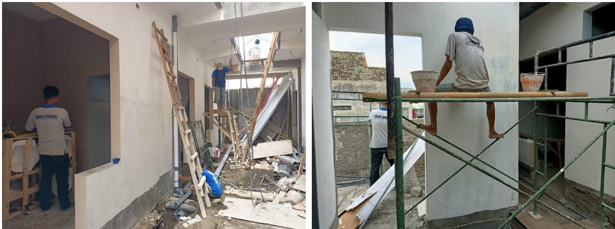
Figure 4. Progress of Boarding House Construction Source: Researcher Process, 2024
